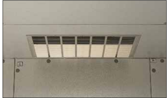
The PRS-2 evaporator grille mounts flush in a standard 4" thick ceiling panel allowing maximum storage space inside the walk-in.
